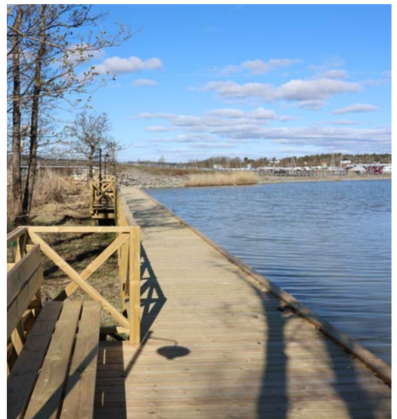
New jetties at Edanö-gård – a perfect stop on a walk or outing.
